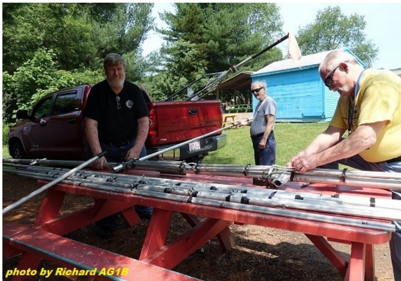
(l-r) Jim N1JCW, Loren N1IQI and Mark KCIACF assembling the beam elements
