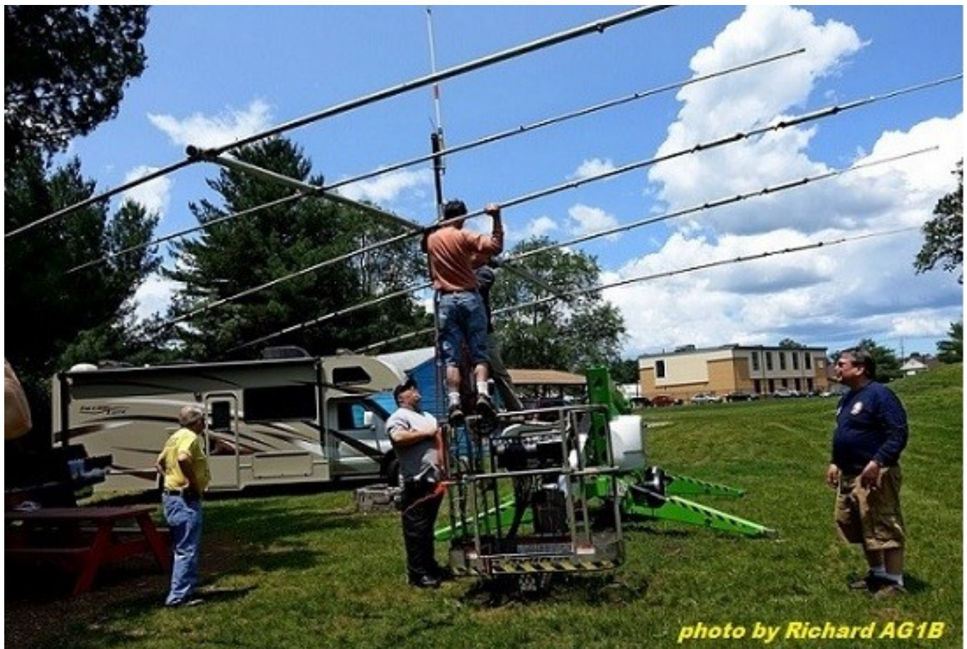
The crew continues to install the beam antenna
