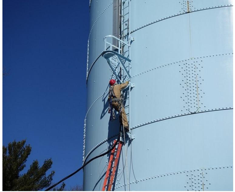
First climber up the ladder
