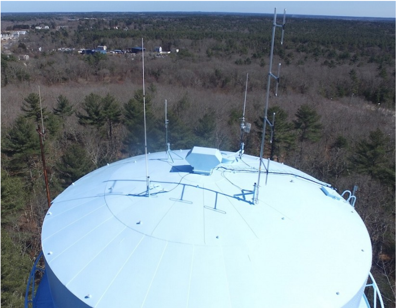
View of the top of the tank after work complete
