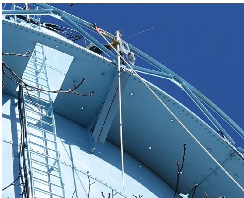
GP9 antenna on the catwalk with crew
