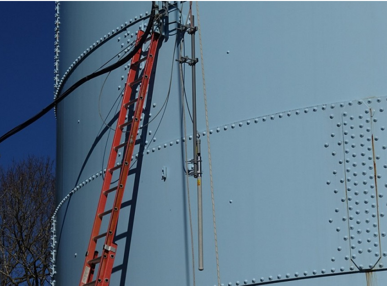
Hoisting the mesh network omni antenna, pole and Ubiquity 2GHZ bullet
