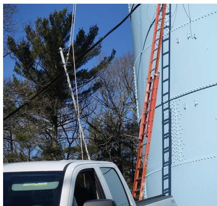
Lowering the black antenna - previously used for .18 transmit
