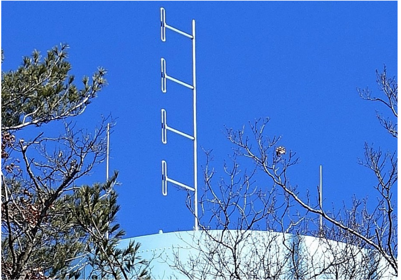
From left to right, Dual Band Comet GP9 (for packet), Sinclair antenna, 70 cm
