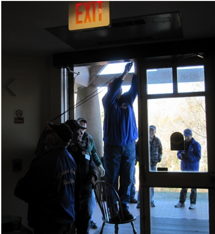
...continue routing the coax into the visitor center... Richard AB1B (our tallest crew member!) up on a chair securing the coax to prevent damage and allow the doors to close normally.
