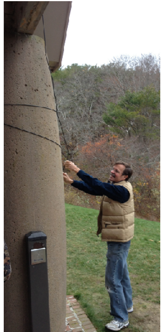
John KB1ODS joins the crew and runs Coax to the R5 vertical
