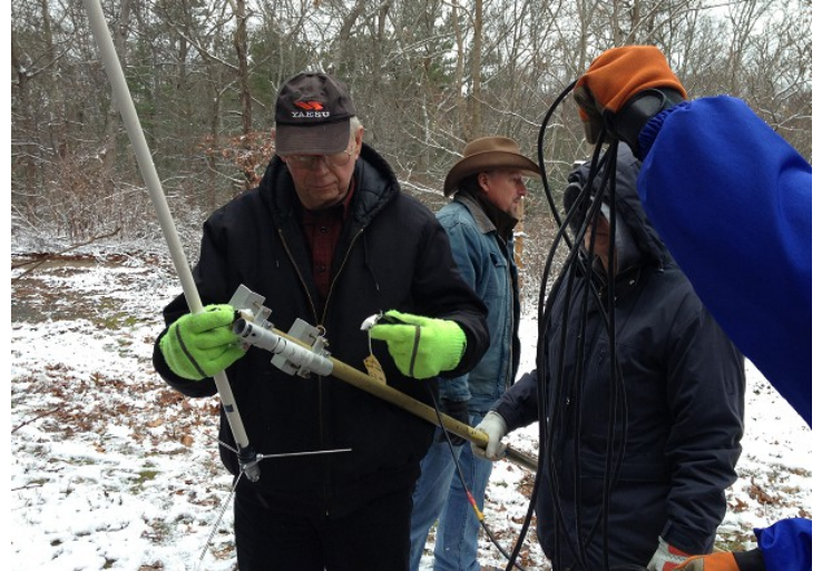
Richard AG1B assembling the 2Meter vertical with help from the team.
