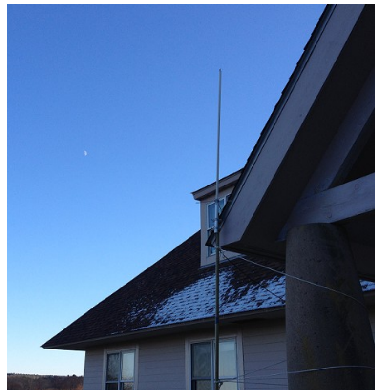
The 2Meter Omni strapped to the back entrance of the Visitor center. (left) The R5 above the back entrance
