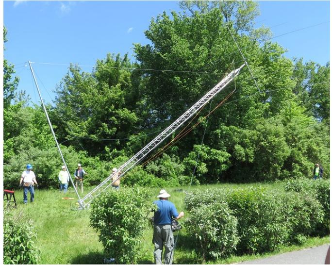
The Beam Team continues to raise the tower using a Falling Derrick system
