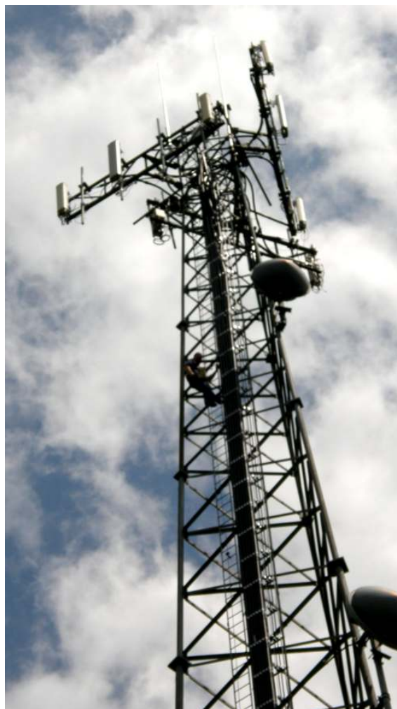
John Baker (JB) climbing the tower
