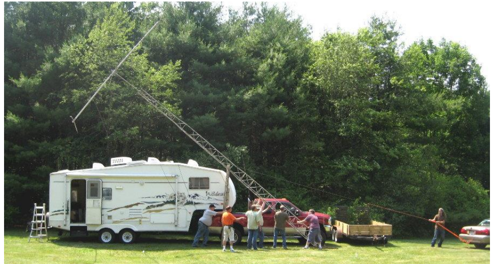
LOWERING THE TOWER: This photo gives you an idea of the height of the tower and size of the beam
