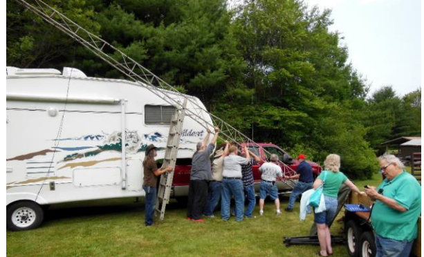
Raising the tower by hand
