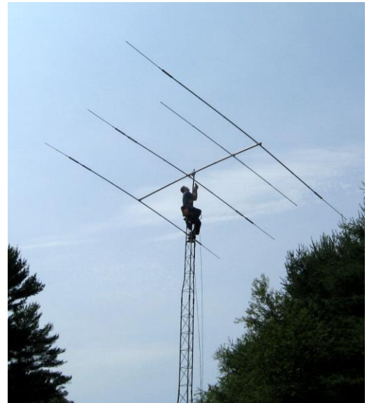
Eric Lewis SWL leveling the beam
