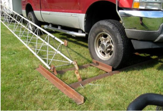
Hinged base and support frame
