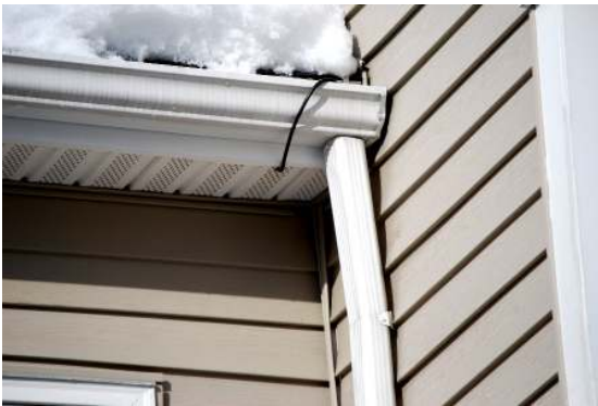
Out through soffit and into gutter downspout
