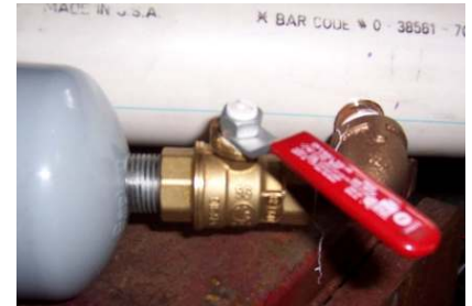
Firing - control valve
