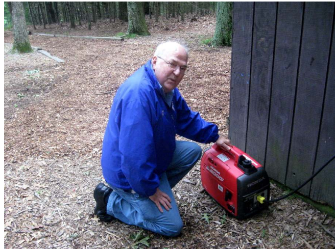
Bruce Hayden N11X inspecting the club's 1000 watt generator
