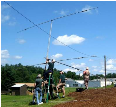
Assembling the Beam Antenna
