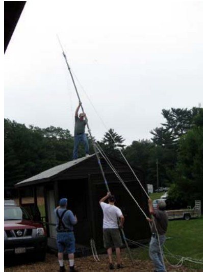
Matt's KB1OSV Antenna Crew Jim Tovet KB1EUI on the roof
