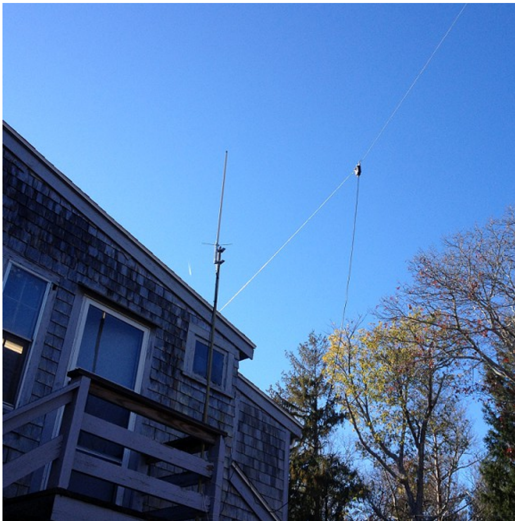
The 40M Window and the 2M vertical at the Admin building
