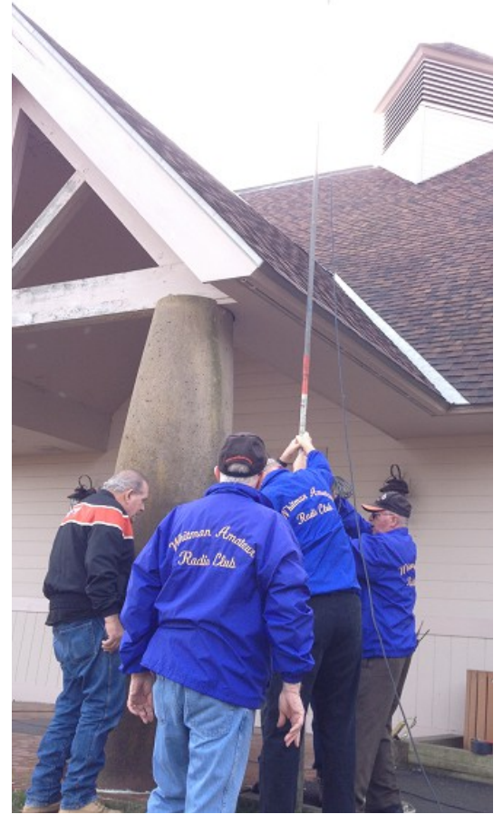
We also assembled a 2 Meter beam atop a 30' painters pole and secured it in place
