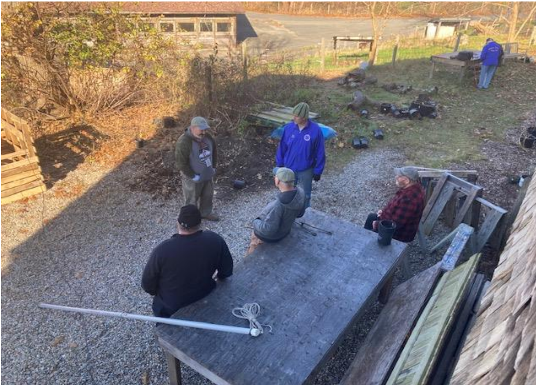
Installing the Antennas at the Horticulture Building
