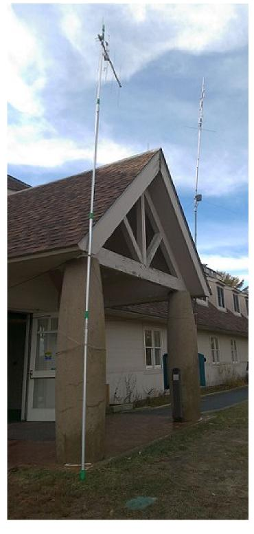
The 2Meter beam was assembled atop the 30' painters pole and also lashed into place.
